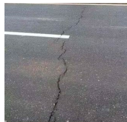
(a) Lateral crack
