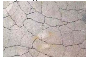
(c) Grid crack
