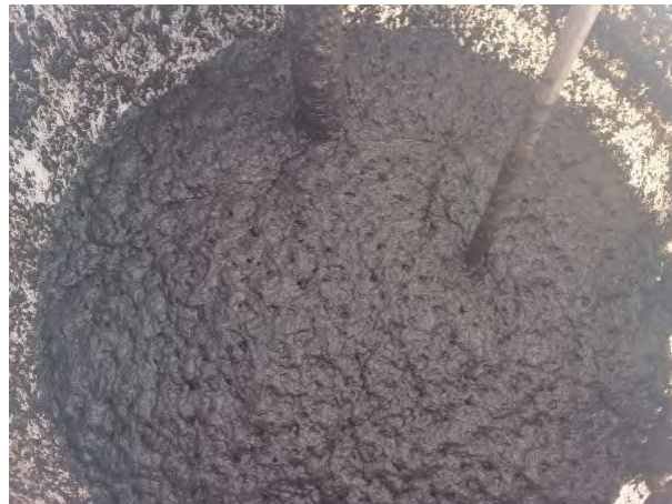
Figure 6 Disposal of flushing fluid and flocculation of broken glue.
