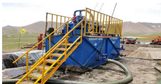
Figure 3: Field test of a 6-6 borehole in the Muli Junan project.
