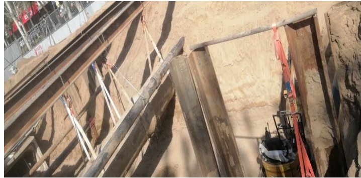
Figure 1: Complex Pipeline Relationships at the Construction Site
