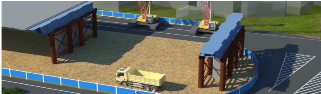
Figure 4: Simulation of Bridge Segment Lifting and Installation
