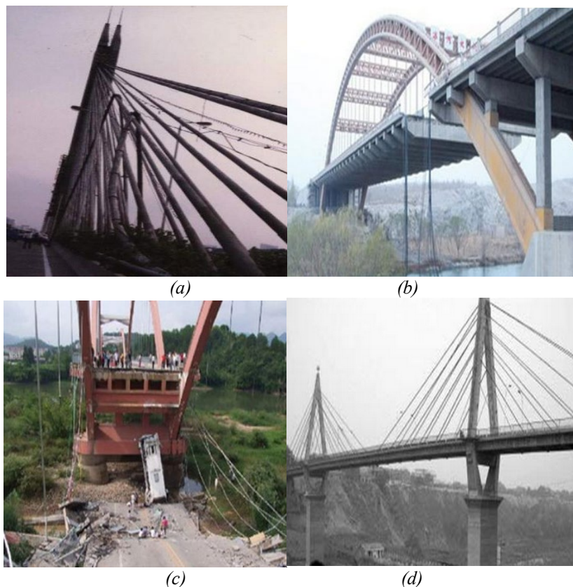
Fig.1 Typical case of damage for cable or suspender of the cable-strut system bridges
