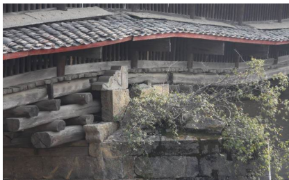
Figure 12: Anhua Shiyi Bridge
