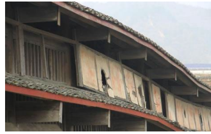
Figure 9: Anhua Shiyi Bridge
