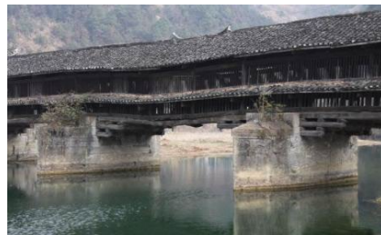
Figure 13: Anhua Fuxing Bridge
