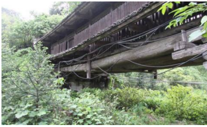
Figure 8: Anhua Wanshan Bridge
