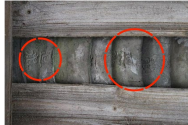
Figure 17: Xinning Huilong Bridge
