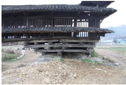
Figure 3: Anhua Xiaojia Bridge
