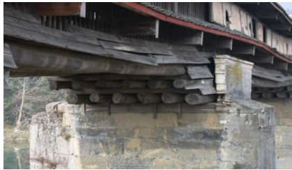
Figure 10: Anhua Shiyi Bridge
