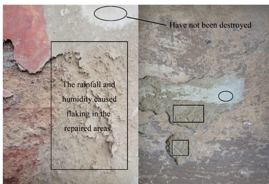
Figure 6 rainfall and humidity caused the repaired materials flaking (left is the 191 st grotto and right is the 59 th grotto)
