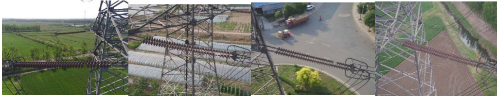
Figure 1: Image of partial insulator defects
